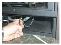
Mount the 3-panel Screen Door / Frame Assembly to the flange on Sub-Frame, ensuring to line-up holes. Secure using the 4 screws provided.
